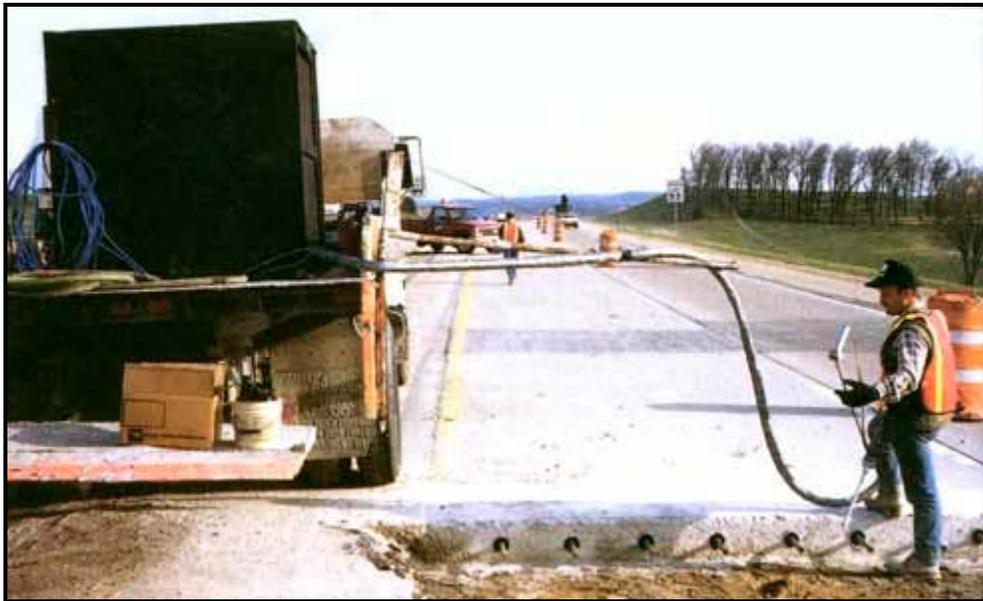
**Dowels must be properly installed to transfer loads at joints and patches**
