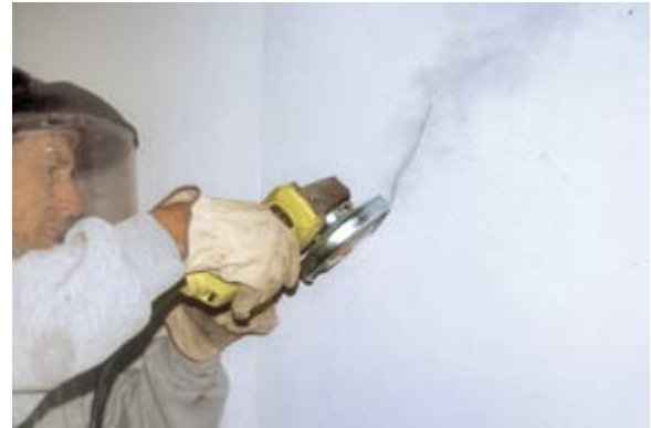
Fig. 6: Chasing the crack with a 4-in. (100-mm) diamond blade to produce a 3/8-in. (10-mm) deep groove
