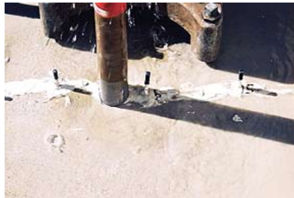
Fig. 23: Cores being taken after completion of injection
