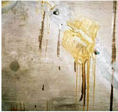
Fig. 10: No problem has so vexed the injection craft as much as leaking seals during injection
