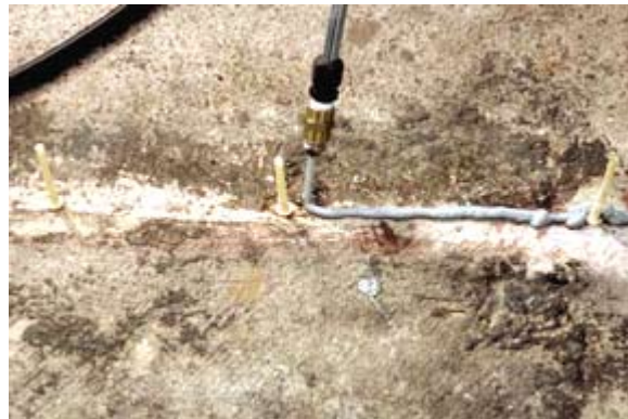
Fig. 17: In contrast, a hydrant can provide fresh, precisely proportioned, and thoroughly mixed seal epoxy
