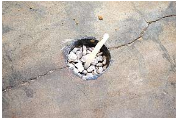
Fig. 20: Clean pea gravel and injection tube are placed in the port, and a stiff epoxy mortar cap is used to seal the top
