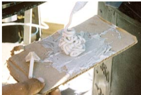
Fig. 17: In contrast, a hydrant can provide fresh, precisely proportioned, and thoroughly mixed seal epoxy
