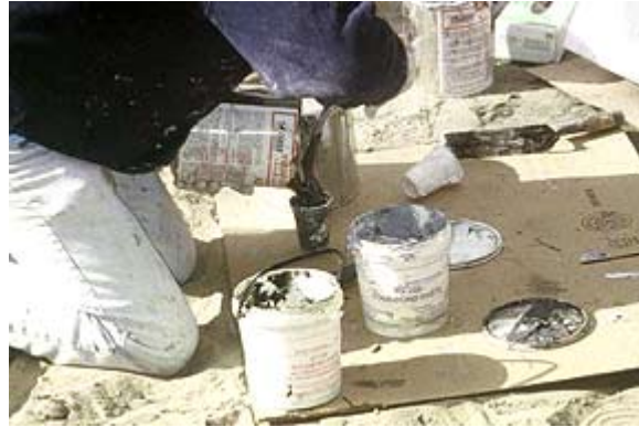
Fig. 16: Manual preparation of resin results in extra cleanup and waste
