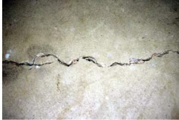
Fig. 2: The width (> 0.088 in. [2.2 mm]) and cleanliness of this crack make it an ideal candidate for packing
