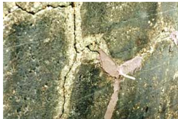
Fig. 14: An insertion port is secured with capping material
