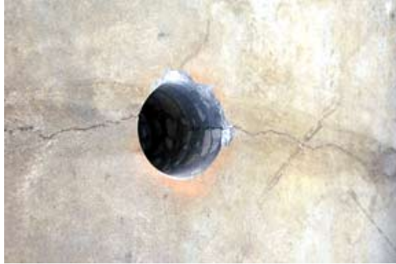
Fig. 19: Two-in. (50-mm) diameter cores work well for master ports
