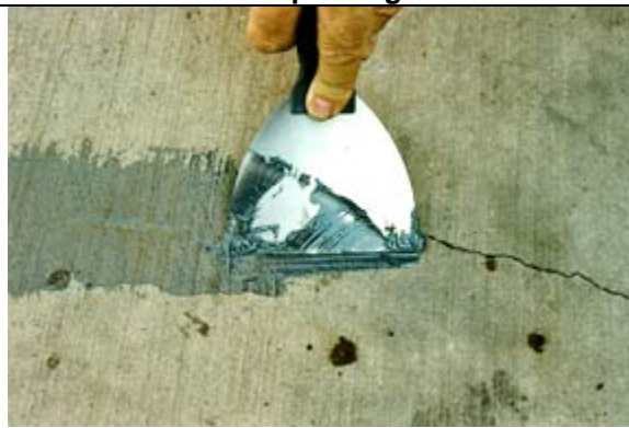
Fig. 2: The width (> 0.088 in. [2.2 mm]) and cleanliness of this crack make it an ideal candidate for packing
