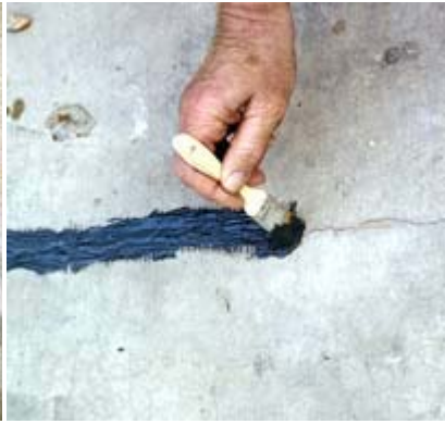
Fig. 11: A stiff-bristled Tampico disposable brush works well for applying the scrub coat
