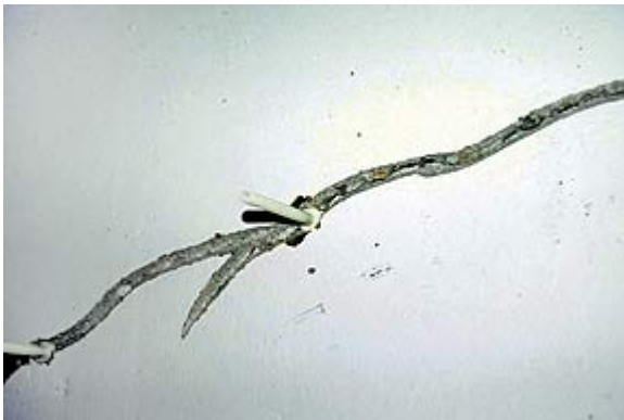
Fig. 8: Ports are installed prior to applying the seal
