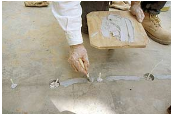
Fig. 20: Clean pea gravel and injection tube are placed in the port, and a stiff epoxy mortar cap is used to seal the top
