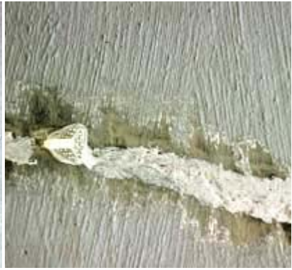
Fig. 12: A typical scrub coat application following porting
