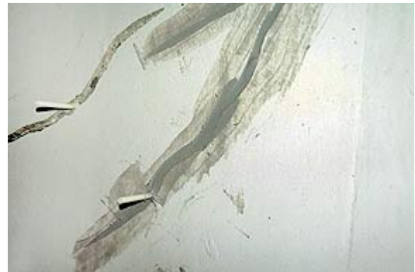
Fig. 6: Chasing the crack with a 4-in. (100-mm) diamond blade to produce a 3/8-in. (10-mm) deep groove
